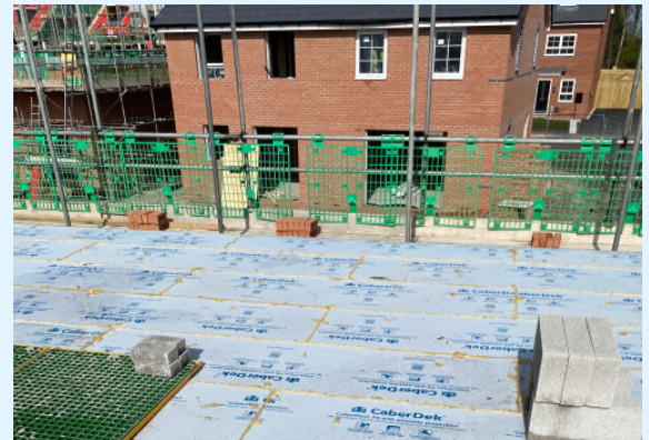
A peel off plastic working platform
