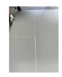
4. Continue installing the panels as required in a staggered pattern by repeating the fixing, and gluing, steps for each panel
