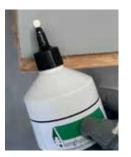
5. Any gaps in the joints and all fixing heads should be sealed with a bead D4 rated PVA tong and groove adhesive or by applying a small area of tape over the head of the fixing
