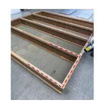
Apply one uninterrupted bead of hybrid polymer joist adhesive to the top of the perimeter joists and noggins corresponding to the area of the first panel to be installed.
