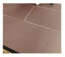
4. Continue installing the panels as required in a staggered pattern by repeating the fixing, gluing, and taping steps for each panel.
