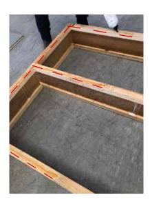
Apply one uninterrupted bead (shown in red) of D4 rated (EN 204) adhesive to the top of the perimeter joists and noggins corresponding to the area of the 1st panel to be installed.
