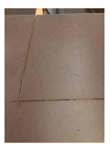
3. Once the perimeter panels are fixed into position with the appropriate mechanical fixings apply the D4 rated (EN 204) adhesive in a continuous bead along the tongue and groove of the joints about to be installed, making sure that the entire joint that is to be fixed is covered.
