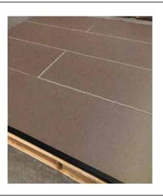
8. Only after the completion of all construction work should the excess adhesive be removed with a hand scraper. Use a soft brush to clean the floor.
