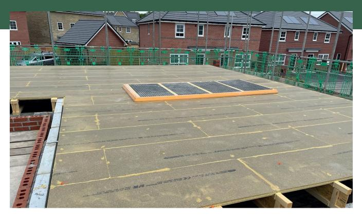
**Longhouse Coating EcoProtect & EcoProtect+** is a new environmentally friendly coating system for P5 grade chipboard and OSB flooring, that enables the construction of a safe slip resistant working platform during the construction process.
